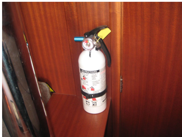
FIGURE 50 – PORTABLE FIRE EXTINGUISHER AT DINING TABLE
