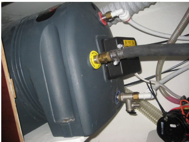
FIGURE 29 – WATER HEATER
