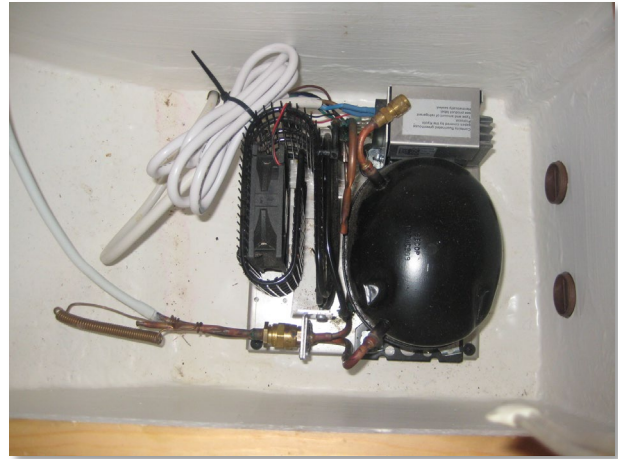
FIGURE 44 – COMPRESSOR UNIT FOR REFRIGERATOR
