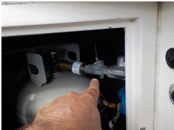
FIGURE 43 – SINGLE STAGE REGULATOR IN UNSUITABLE PROPANE LOCKER
