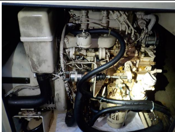
FIGURE 29 - GENERATOR INSTALLATION IN ENGINE SPACE
