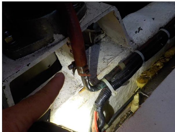
FIGURE 44 – IMPROPER FUEL HOSE CONNECTION AT PORT MAIN ENGINE
