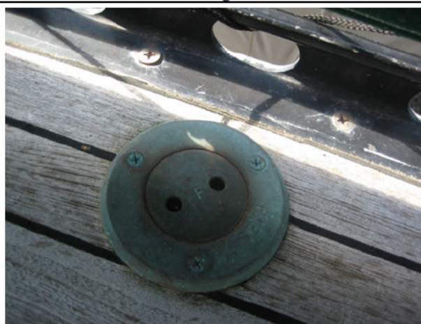
FIGURE 26 – DECK FILL PORT SIDE DECK
