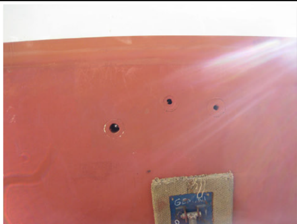
FIGURE 33 – THROUGH-HULLS PORT SIDE
