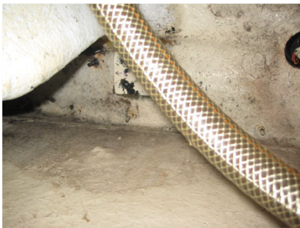
FIGURE 13 - HULL/DECK JOINT IN FOREPEAK RODE LOCKER
