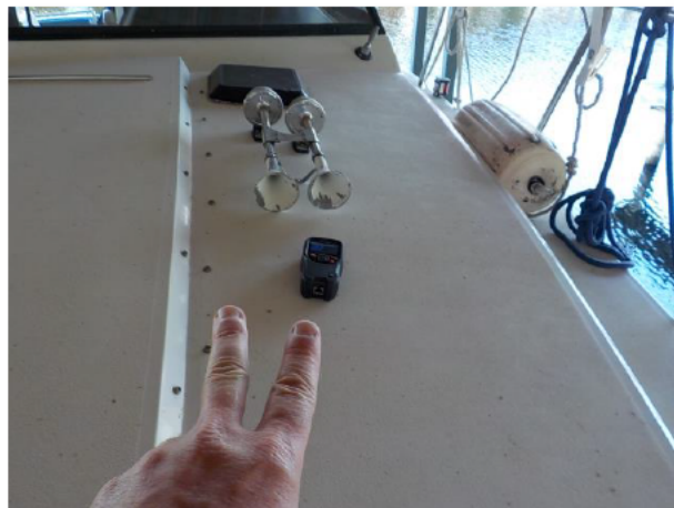
FIGURE 38 – ELEVATED MOISTURE OBSERVED ON FOREDECK
